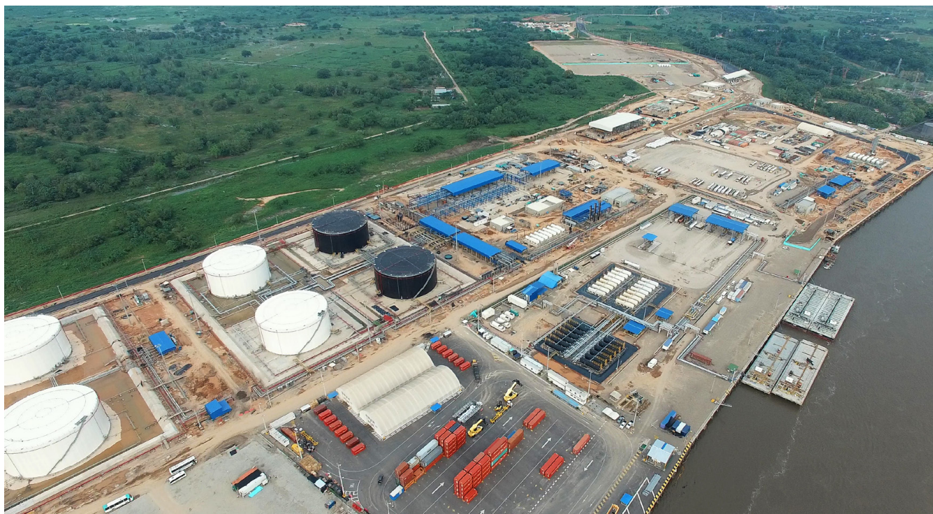
Impala Terminal's inland riverside port on the Magdalena River at Barrancabermeja, Colombia.
